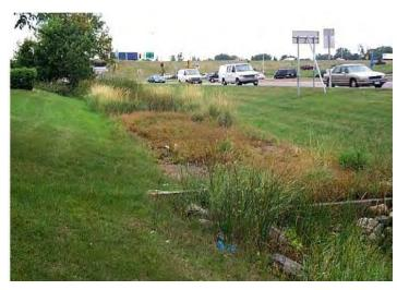
Figure B.13 – Photograph of water quality swale
