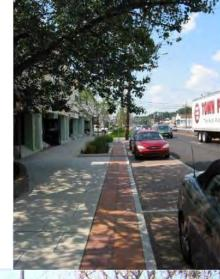
Figure B.9 – Photographs of porous pavement
