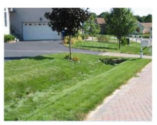
Figure B.12—Photograph of vegetated drainage ways.
