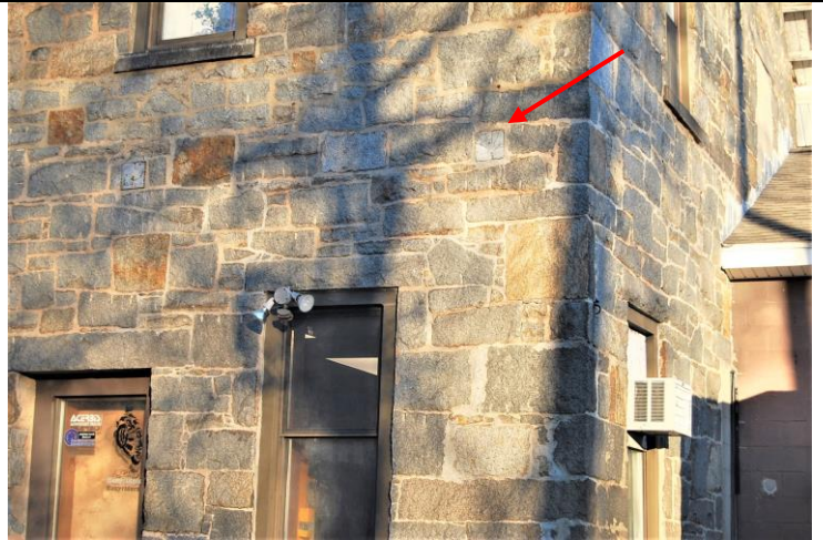
Detail. Stonework and wood nailers where shelter was attached.
