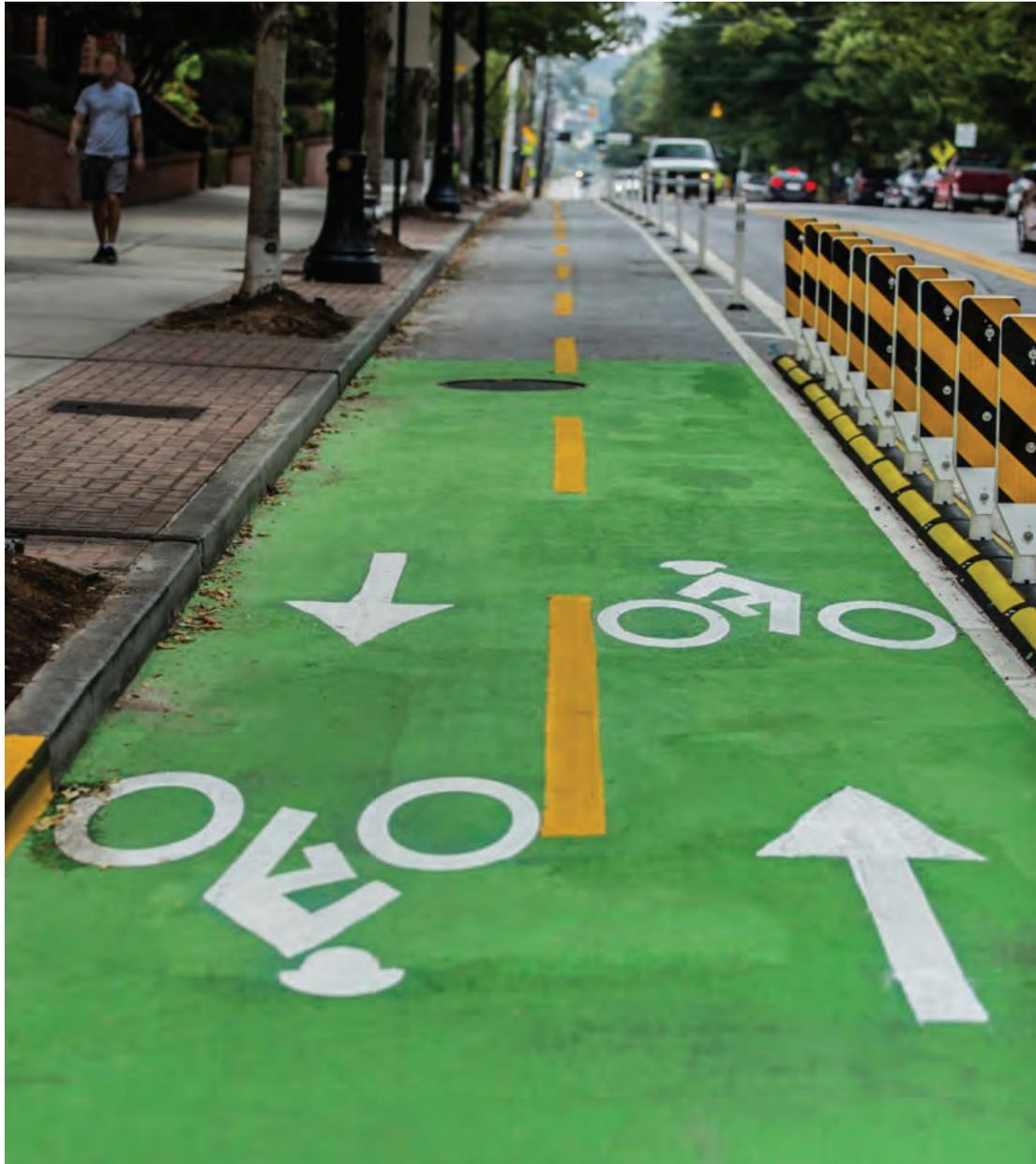
Figure 10-12. A two-way on-street cycle track installed in Jersey City NJ has not only provided space for micro-mobility device users, it has also helped diet a busy arterial to reduce speeds and improve walk safety.
