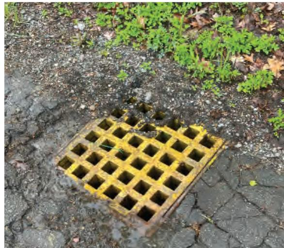
Figure 2-20. Catch basin draining to wetlands with no buffer
