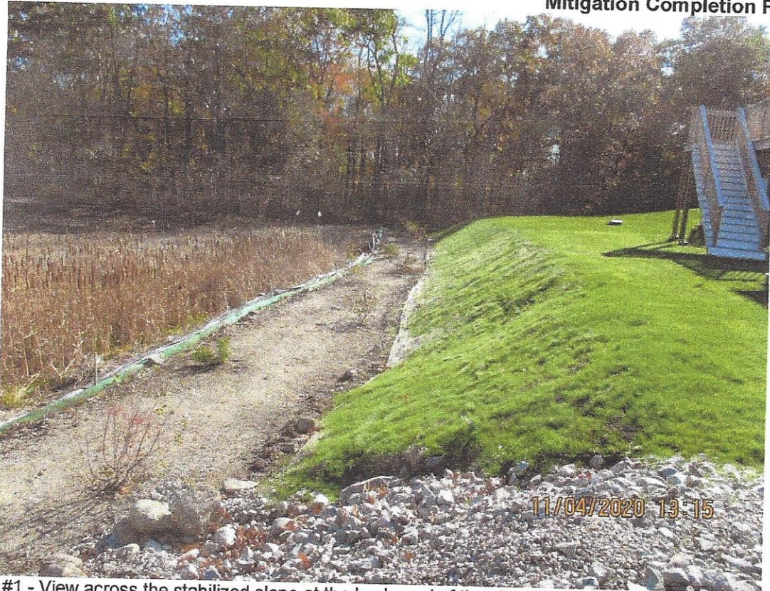
Photograph #1 - View across the stabilized slope at the back yard of the site, which was covered with jute netting and planted with seedlings of shrubs and herbaceous plants. Notice the planting strip along the base of the slope.
