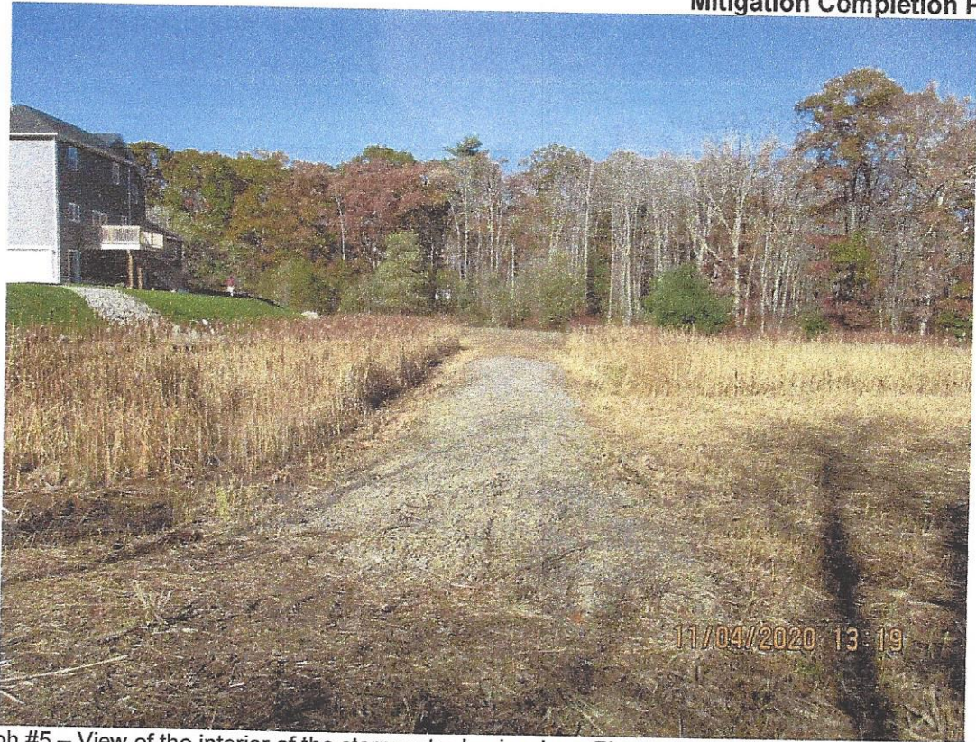
Photograph #5 – View of the interior of the stormwater basin where Phragmites was removed and the stone berm recovered.
